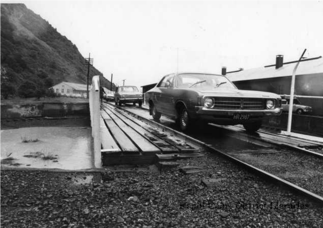
1979 floods – SH1 traffic diverting through rail yards and across the turntable
