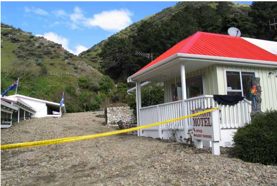
Debris flood through motel
