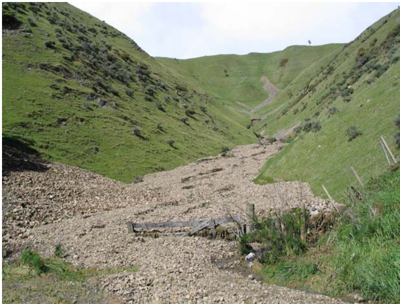
Figure 15. A closer view of Site 7 showing gravel trapped behind the fence and gate above the road. There was, however, little damage to the fence and gate, which suggests that the gravel accumulated slowly, from a hyper-concentrated debris flood of water laden with silt, sand, and gravel. Most of the finer sediment was carried away in the flood water. This type of mechanism shows that steel catch fences above the road could be used effectively to control future debris floods.
