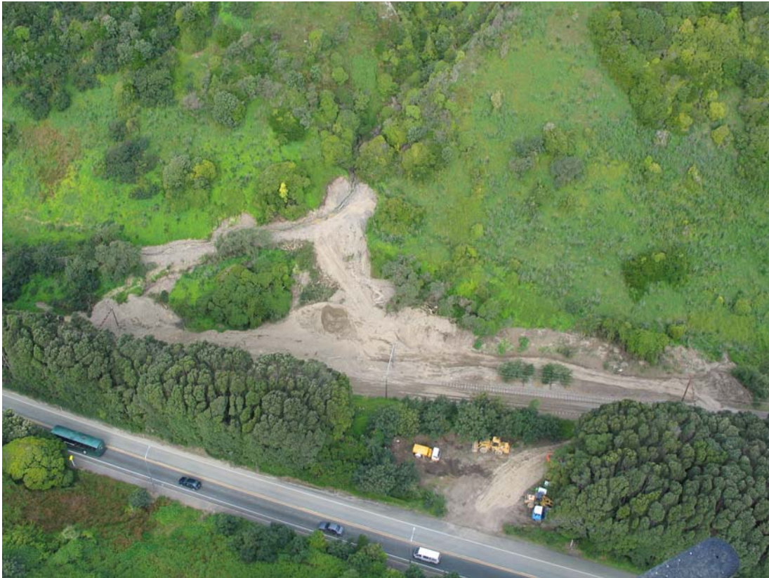
Figure 18. Aerial view of damage at Sites 8 at the bottom of the ‘Hill Road Gully’ on Wednesday 8 October showing the large volume of gravel, sand and silt that spilled across the NIMT railway line during the 3 October flood. Control of debris higher up this gully would minimise problems at this site. Some form of debris passing structure may also be necessary at the culvert entrance to prevent blockages and allow flood water to be safely passed under the railway and SH 1.
