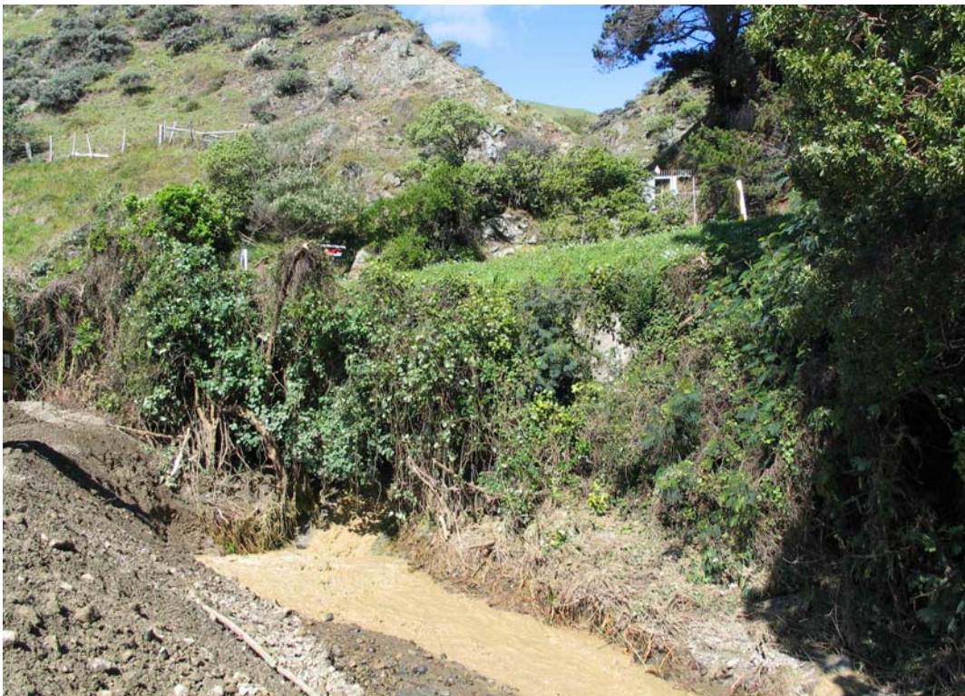
Figure 6. Culvert discharge area behind the Belvedere Motel the day after the flood. This view shows that vegetation above the culvert on the side of the hill road was unaffected by the flood, indicating that all the gravel and flood water passed through the culvert and not over the road.
